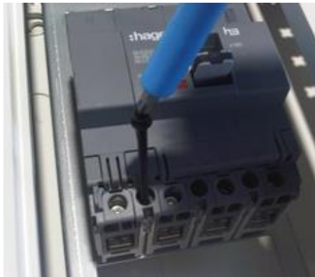
MCCB fixing on metal plate with M4 screws delivered-by
