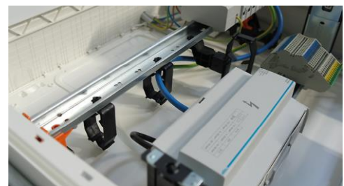
Mounting example in flush high-depth
