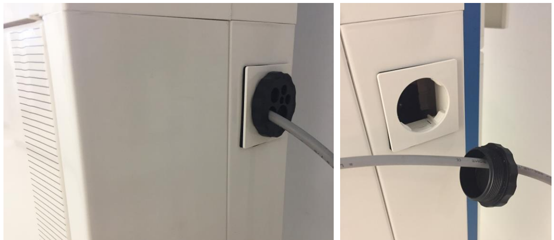
FD00P6 mounting into New VegaD surface board
