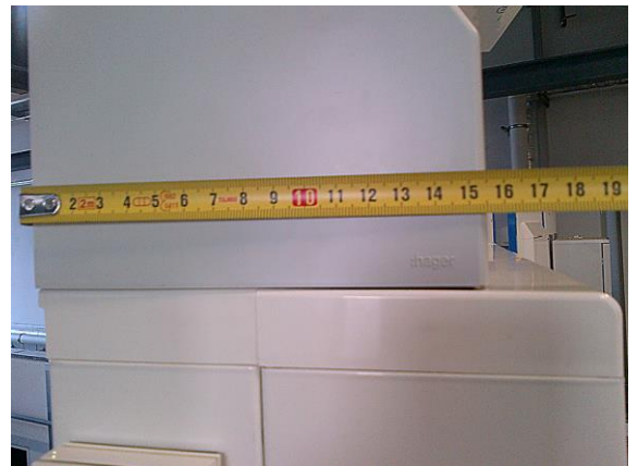
Cross section [mm] 155 x 195 or 195 x 155
