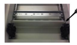
Direct screw connection on the mounting rails
