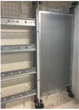
Installation of UZ40F1 in FWB distribution board, size 42: Installation from the front
