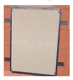
Plaster guard inserted into the wall cabinet with pre-punched holes
