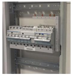
Partition FWU00Vx also compatible with the vertical KCL... busbar system
