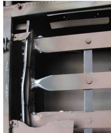
Significant damage to system with high subsequent costs following an arc fault.
