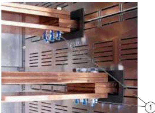
Example of marking screw connections
