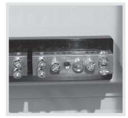
Remove Copper Bridge and centre screw as shown above
