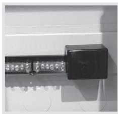
Use the vacant screw hole to insert the Meter Neutral Seal.
