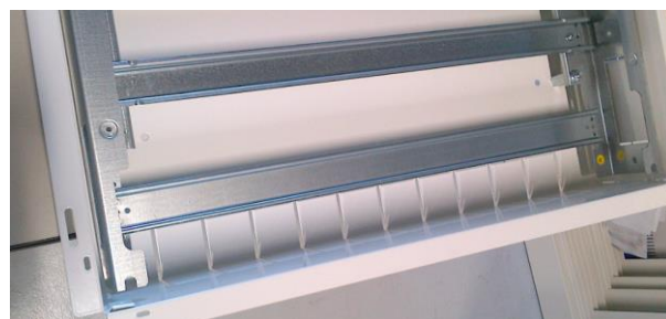
Mounting of the 24 modules DIN rail FZ24D in the board FW424FT
