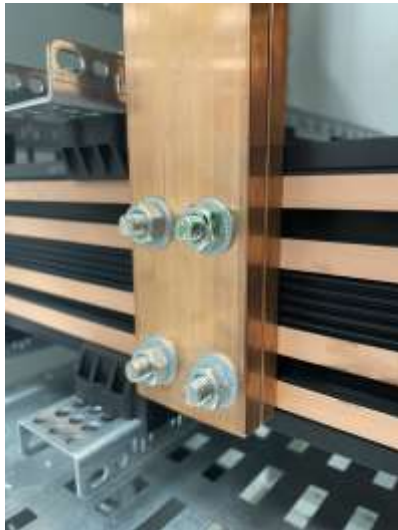
Example of connection up to 1600 A
