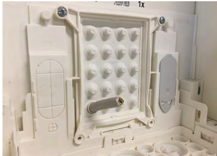
Flange FZ428 installed on the rear of the cabinet
